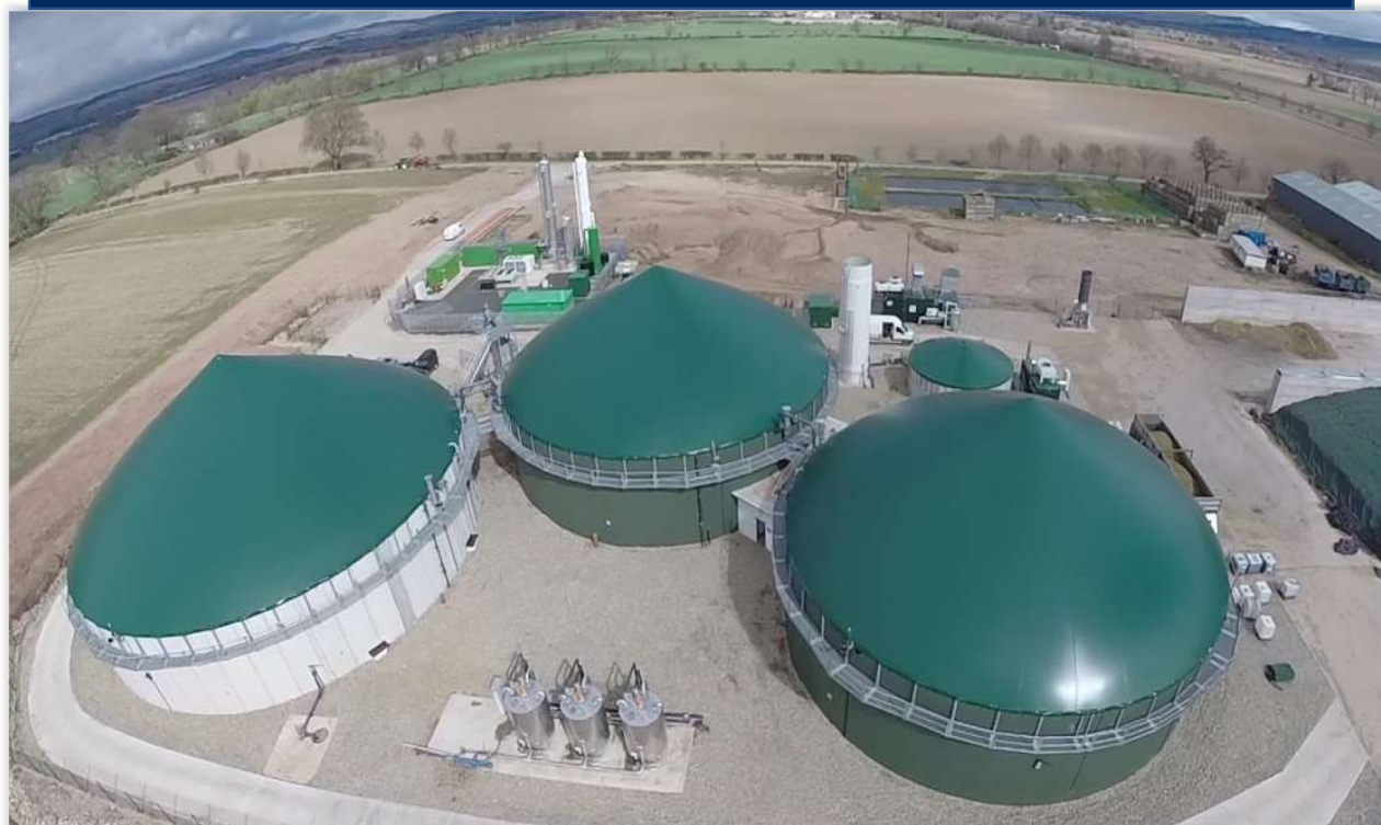
Biomethane Plant in Coupar Angus, Perth (Scotland)
