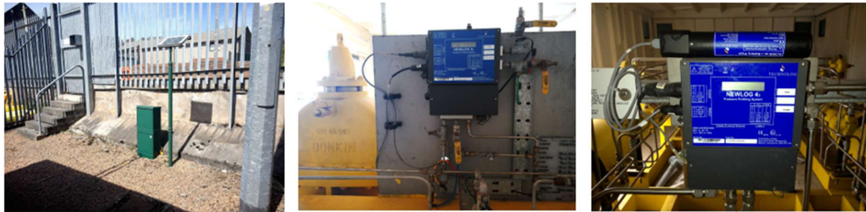
Figure 34: Solar panel trial on profiling governor station in Dundee
